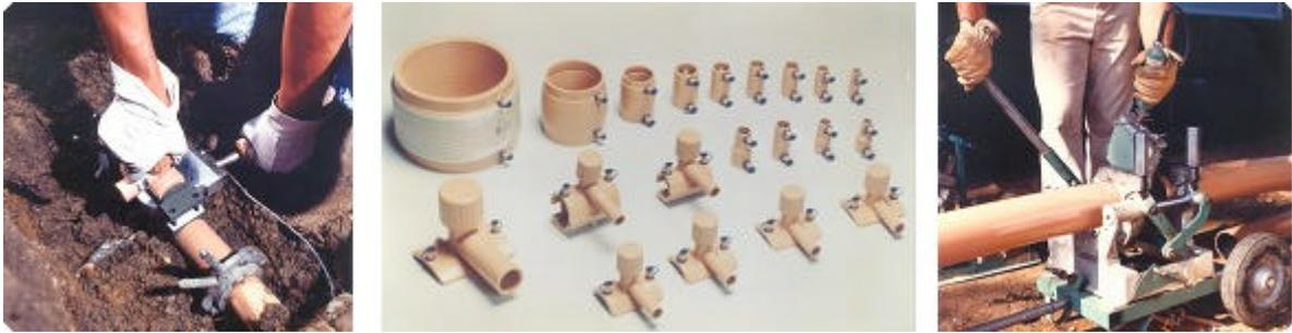
When polyethylene pipes were first introduced to the United Kingdom, in 1969, they were supplied in imperial dimensions. The use of these pipes continued until 1977, after which the gas industry completed the conversion to metric pipe dimensions. The table below shows the dimensions of the pipes which were supplied.
