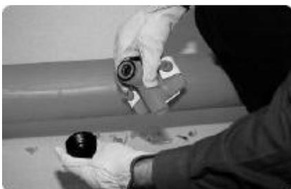
d. Remove the fitting from its packaging and then remove the cap to expose the top of the integral cutter which should be flush with the top of the fitting.
