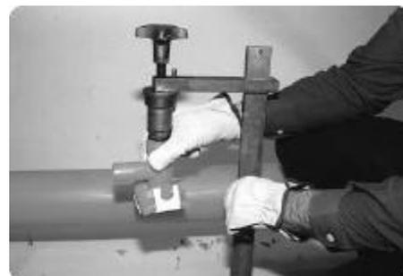
f. Remove the cardboard protector from the base of the tapping tee and position the fitting onto the previously prepared area of the pipe. Secure the top loading clamp and apply the correct top load of between 1kN and 1.5kN in accordance with the manufacturers instructions for the style of clamp being used. During the latter two steps, it is imperative to ensure that the scraped pipe surface and the fusion pad of the tapping tee are kept clean, dry and free from contamination.
